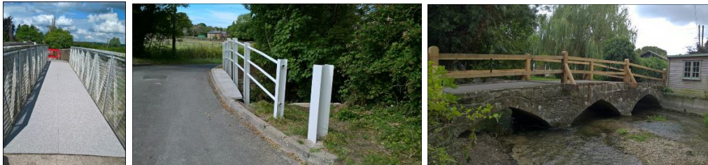
Bridge repairs and renewal was carried out on various types of bridges
