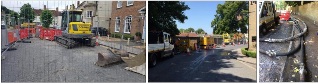
Drainage repairs in Wilton were co-ordinated with works by public utilities
