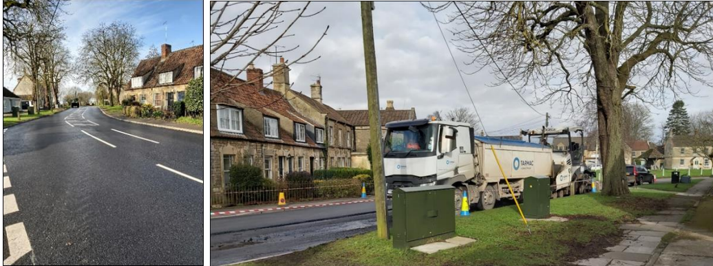
Tarmac resurfacing work continued through the lockdowns to ensure safe delivery of the road resurfacing programme
