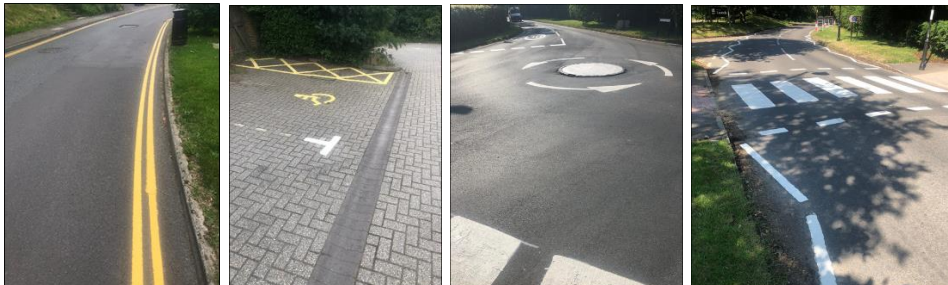
A programme of lining renewal took place during the summer
